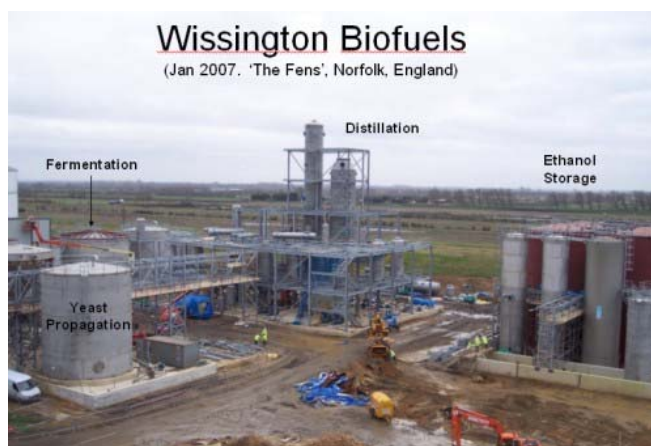
British Sugar bioethanol plant under construction at Wissington Sugar Factory, UK
