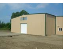
Processing facility and storage freezer addition with capacity for 10 million willow cuttings.
